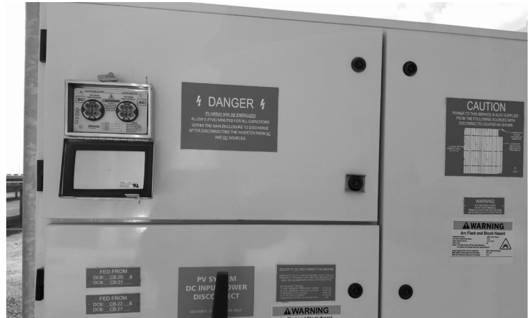
Two Safe-Test Points™ in Stainless Steel housing used to verify the absence of voltage on Line and Load side (DC/AC) of an inverter system in a PV solar application.
