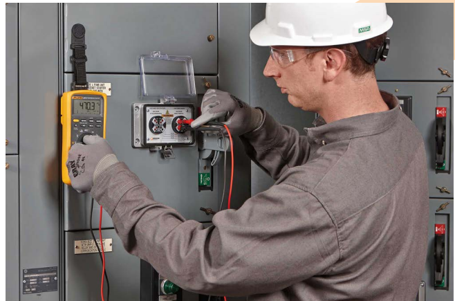
Figure 2: The Voltage Test Station is designed to verify both the presence and absence of voltage from outside the door
